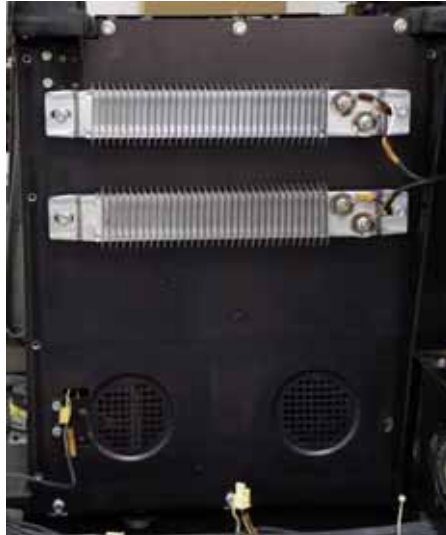
Figure 459: Opening the chamber heater cover
