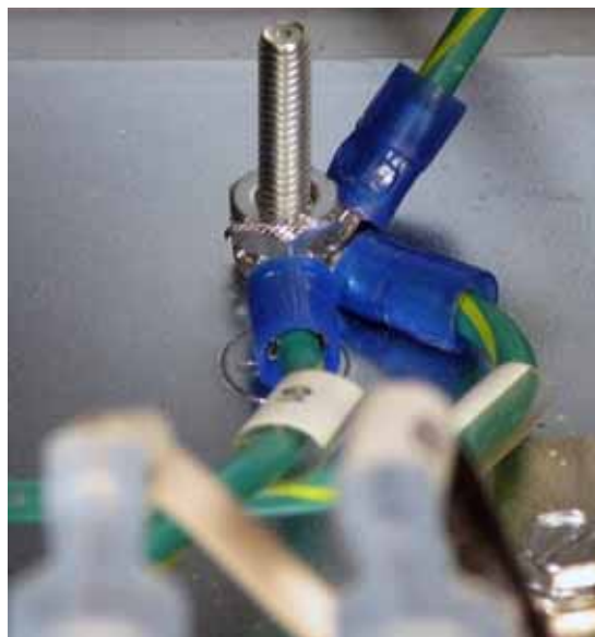
Figure 205: Ground post location
