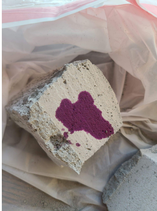
Fig 1: Untreated sample tested with phenolphthalein shows ongoing carbonation
