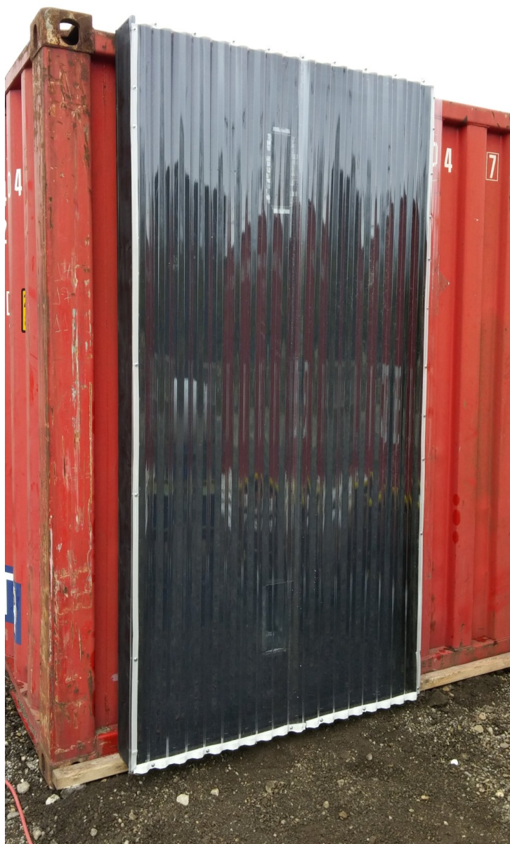
Two corrugated panels, attached on all edges and about to be "stitched" together.
