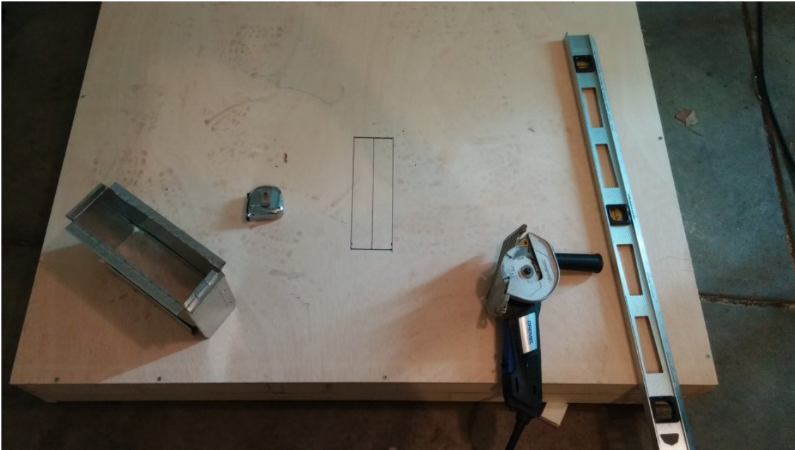
A vent hole, marked and ready to cut.
