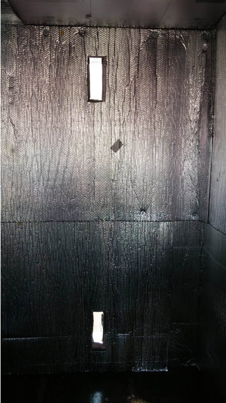
A view from the inside of the container, once the unit is installed and with the inside insulation and reflective barrier in-place.
