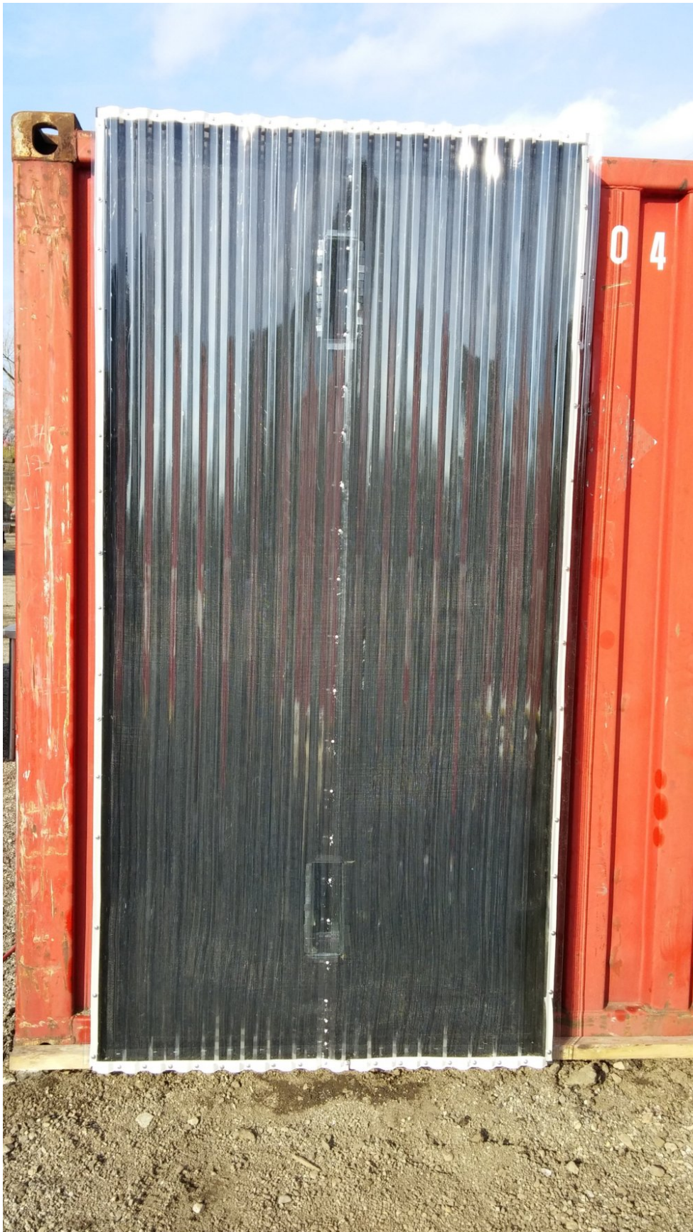
The two panels stitched together with about 20 rivets.
