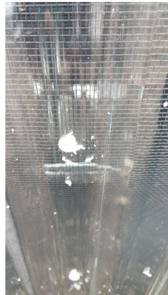
A bad closeup showing a few of the rivets.
