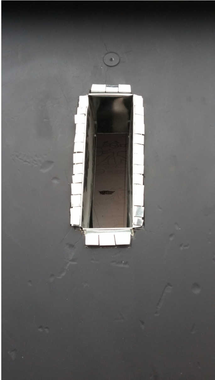
The upper vent.
