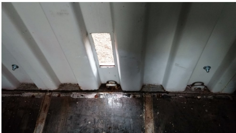
The lower vent hole with mounting holes (bolts
