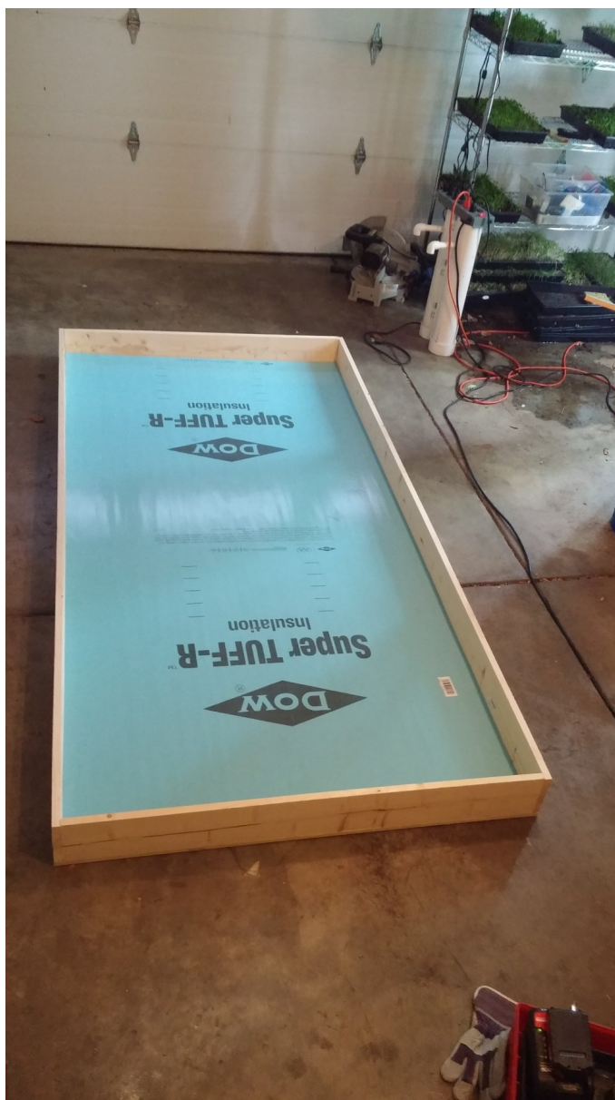
The insulated box frame.
