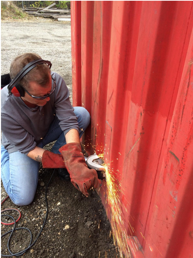
Cutting the lower vent hole.
