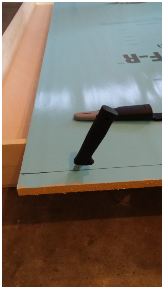
Trimming the insulation
