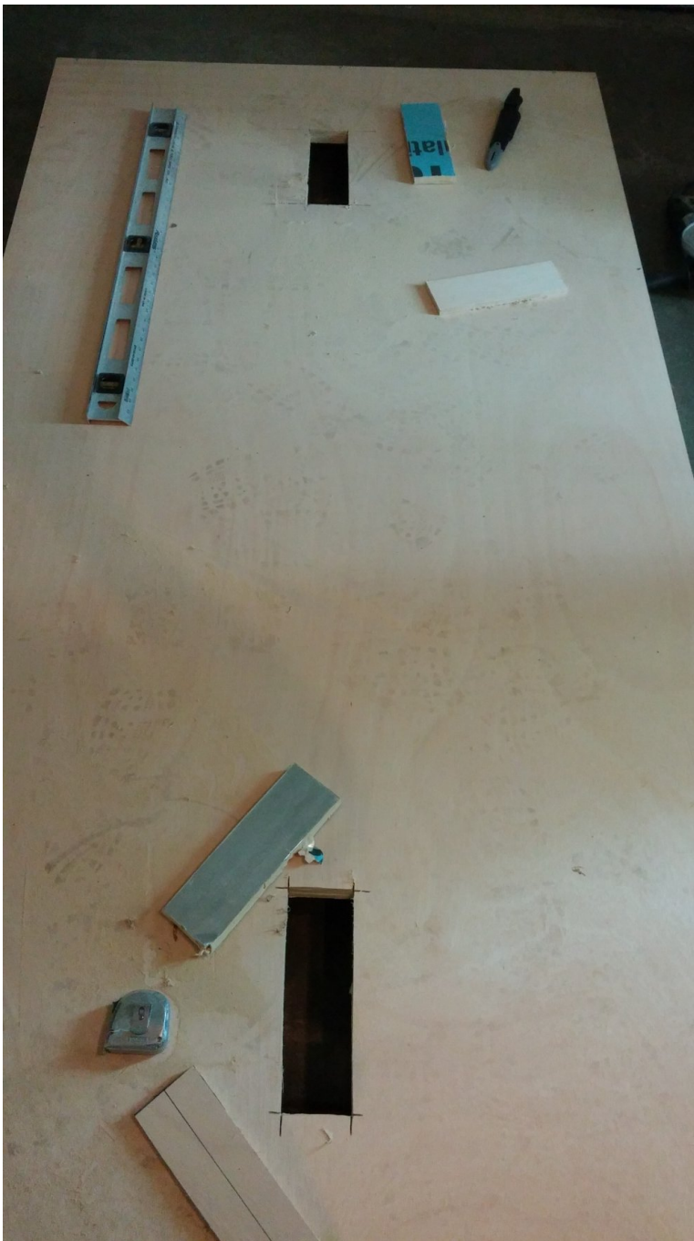
Both vent holes cut out.
